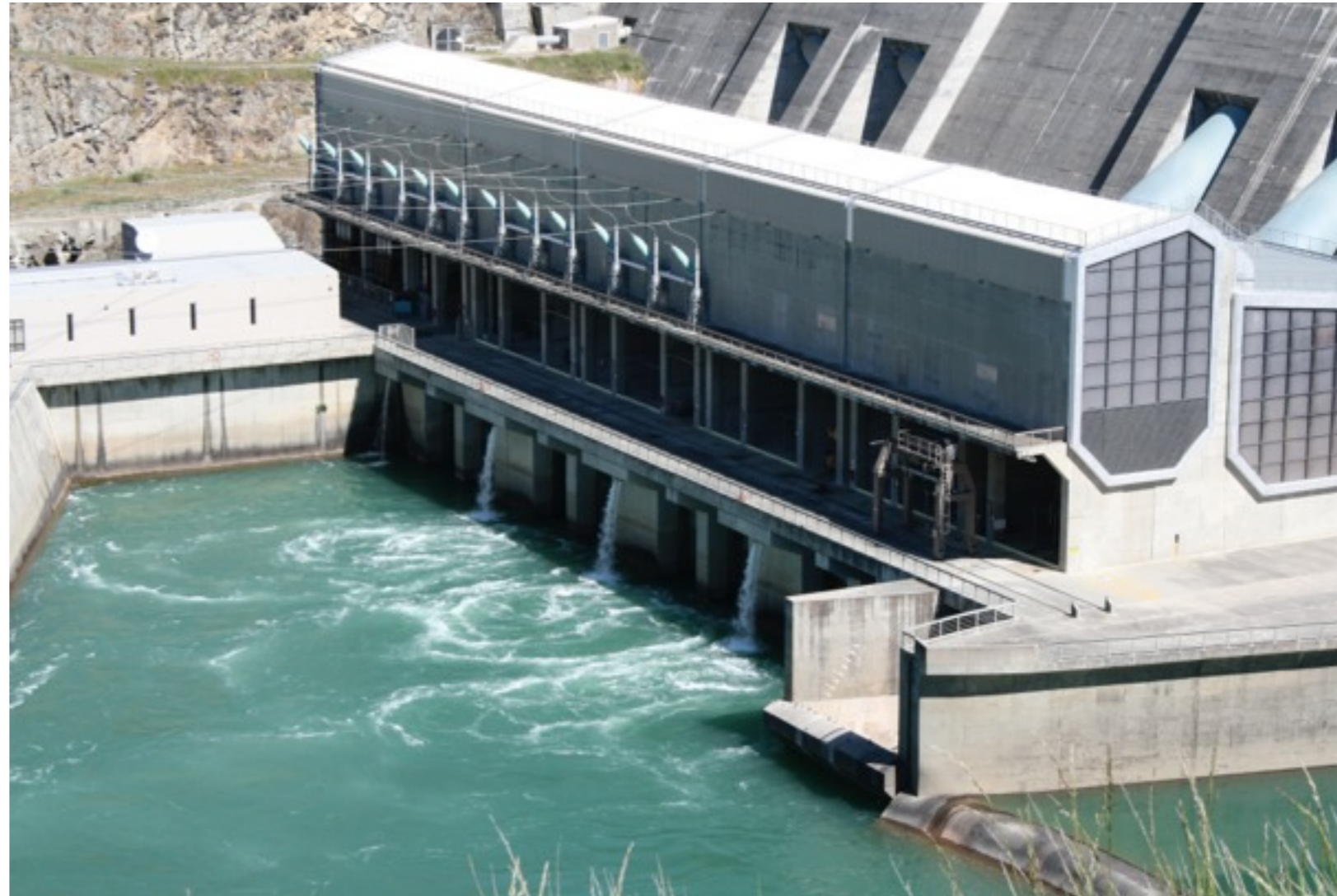
A small hydro-electric power station - Clyde Dam, New Zealand.
